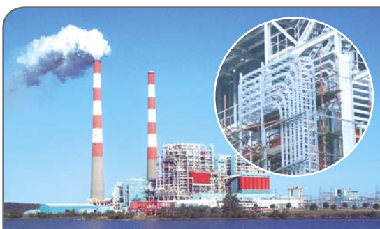
Energy Power Plants
